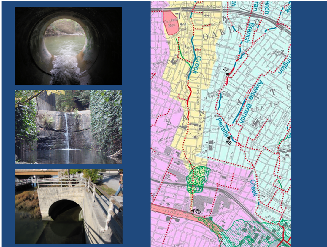
Figure 17. Rainbow trout are prevented from venturing too far upstream or downstream by human-made structures including (counterclockwise from top left): a road culvert under El Centro Avenue; a drop structure at Barry Place; and a large culvert at the Oakland Estuary. The map depicts the lower fragmented reaches of Sausal Creek (left side of figure) where the creek was “channelized” (solid red line), “undergrounded” (dotted red line), not channelized but modified with stormwater infrastructure (blue line), and historical wetland features (green line).
