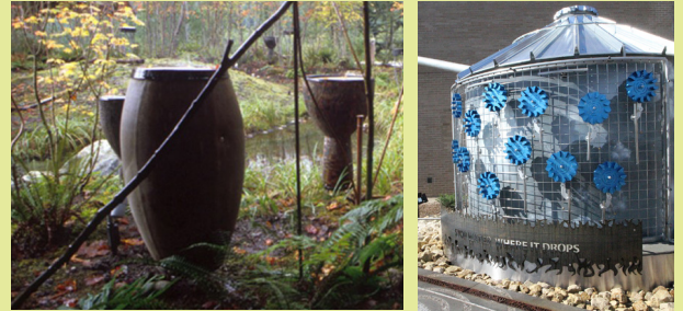
C2: Example rain drum (left) and water storage tanks (right) to collect roof water at Josie de la Cruz Park
