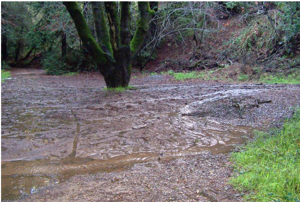
Figure Q: Erosion site #2. Lack of a culverted stream crossing causes water to flow down Sunset Loop Trail, eroding the trail and creating a pile of mud on Sunset Trail (bottom) and in Palo Seco Creek.
