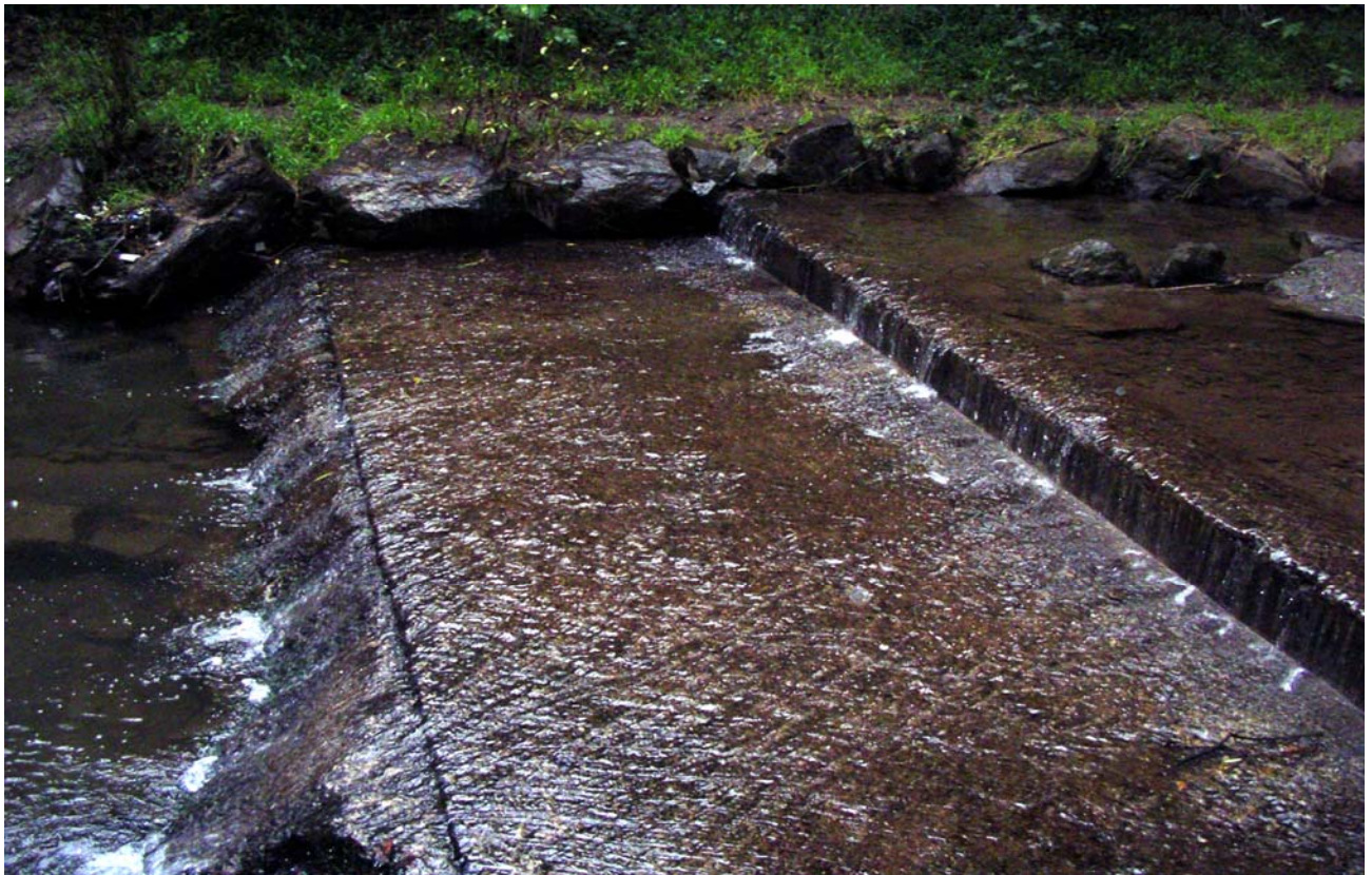
Figure M: These photos are examples of the drop structures in Sausal Creek (SC1) in Dimond Canyon.
