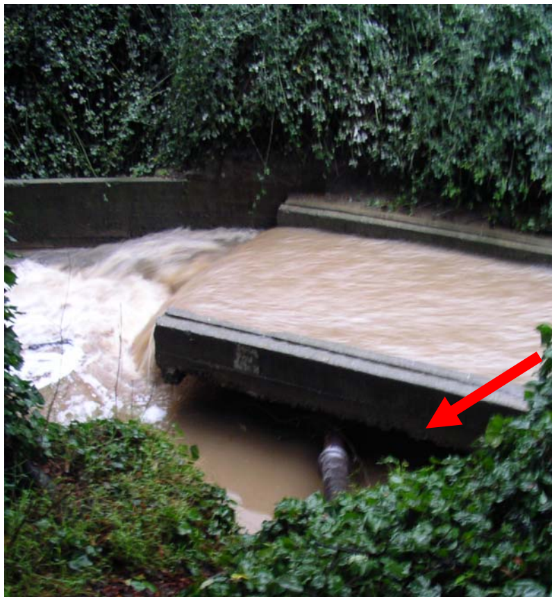
Figure 108: Top: main sewer line in the bed of Sausal Creek This new pipe was installed during the creek restoration in 2001. Bottom: Sausal Creek in Dimond Park. A lateral sewer line is visible underneath the concrete apron (red arrow).
