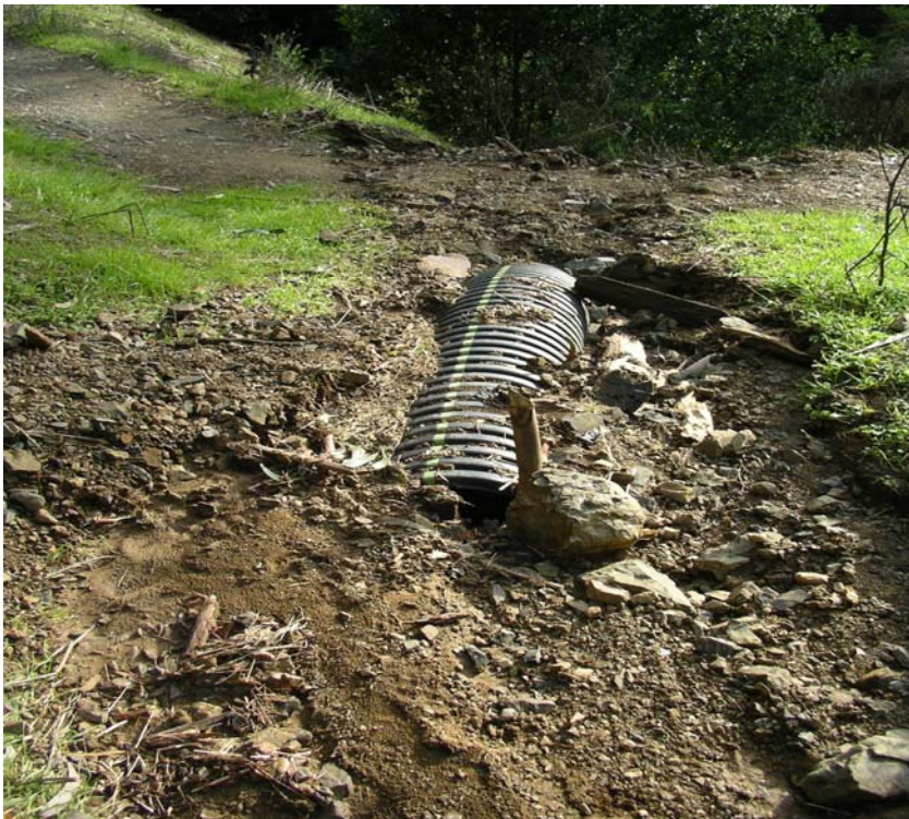
Figure 99: Two examples of ineffective trail crossing repairs. Plastic pipes are too small and can easily clog; both are not placed in the crossing at the proper angle, and are not covered with enough soil to avoid damage. Top: Ineffective repair to trail crossing creek in Joaquin Miller Park. Bottom: Creek can easily flow over trail in higher water events and erode soil and pollute Palo Seco Creek.
