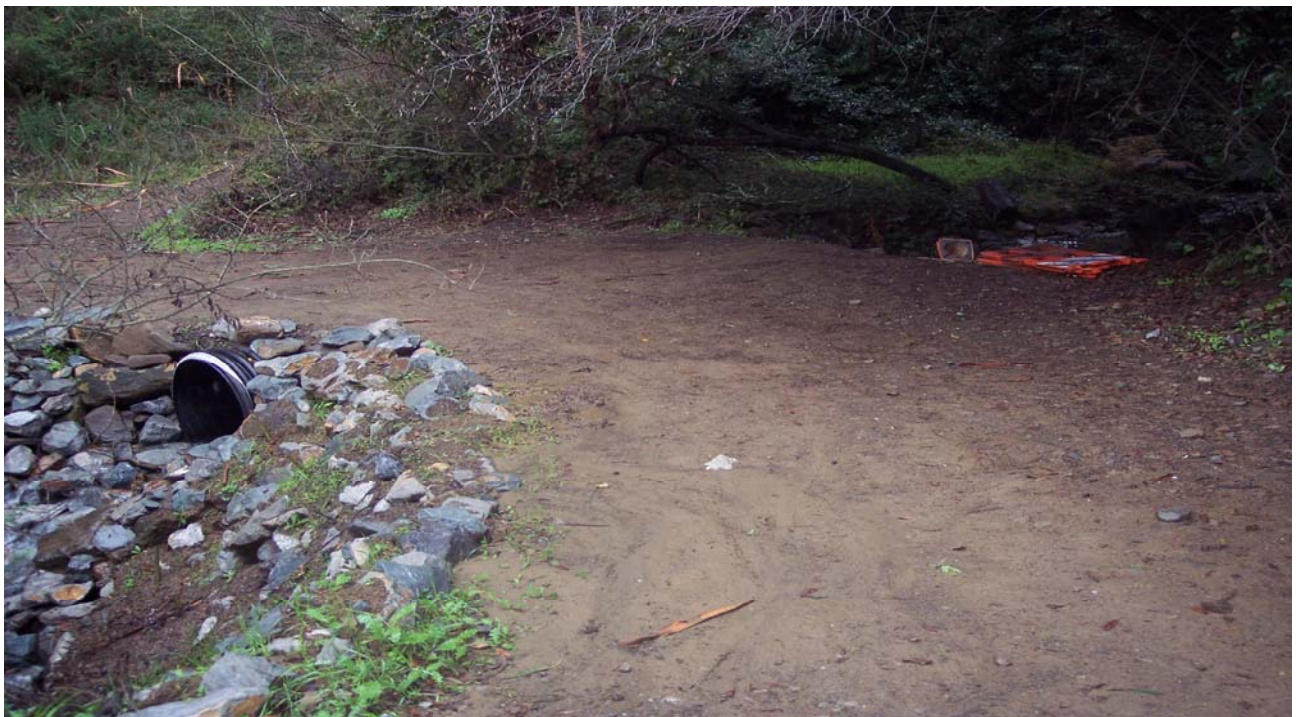
Figure 93: Top: Cinderella Creek with culverted crossing at Sunset Trail erodes and overflows the culvert. Stormwater from the Chabot Space and Science Center has increased the volume of flow in Cinderella creek, increasing erosion. Bottom: Repair in 2007 was done incorrectly by setting the culvert at a flat angle; the proper method is to set the culvert at the slope of the creek bed to reduce downstream erosion. Culvert is also undersized and continues to be overwhelmed by storm flows.
