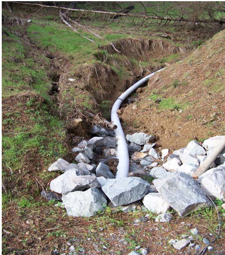
Figure 96: One of many temporary and ineffective repair projects done at Castle Drive erosion site.
