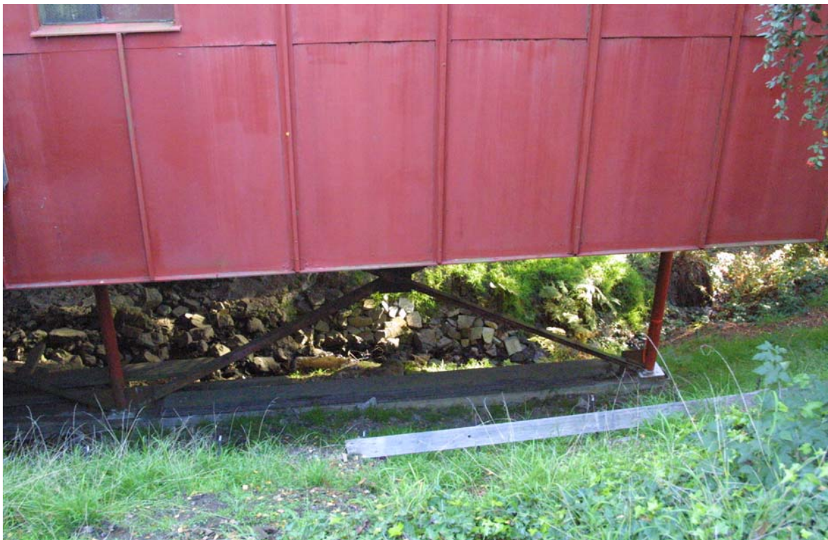
Figure 87: Ephemeral creek channels adjacent and under house with signs of erosion likely from increased volumes of runoff from urbanization of upper Sausal Creek watershed.
