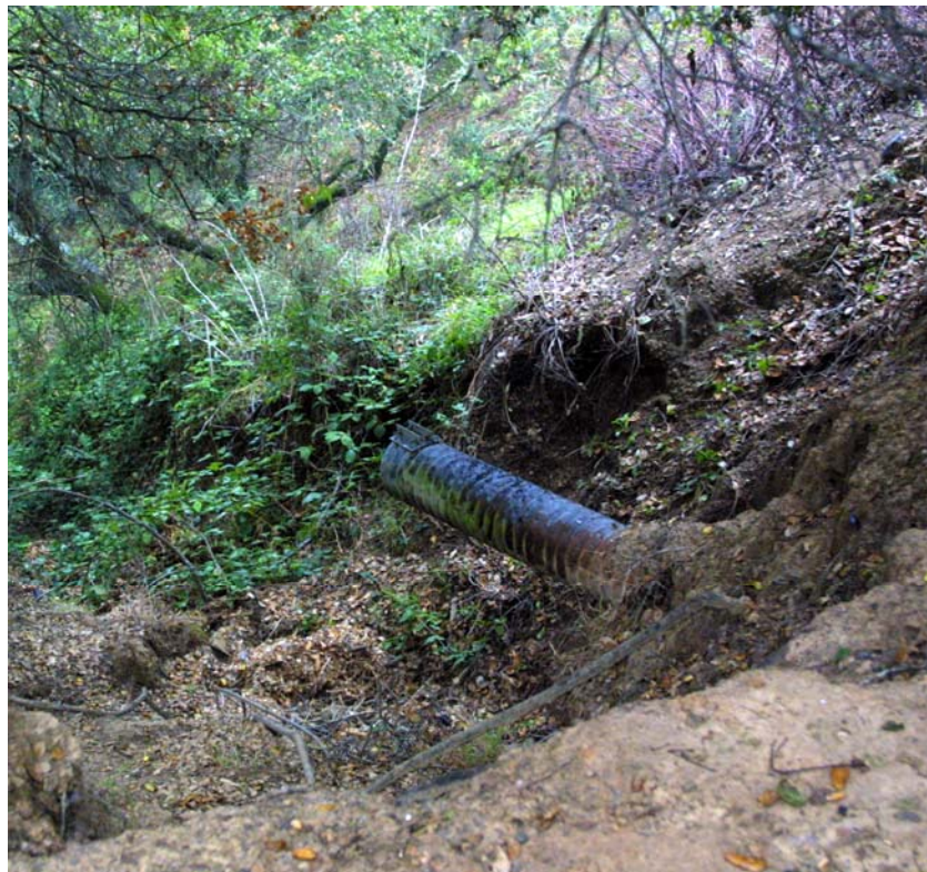
Figure 88: Top: Erosion of ephemeral creek from urban runoff in upper Sausal Creek watershed. Bottom: Erosion from storm drain outlet.
