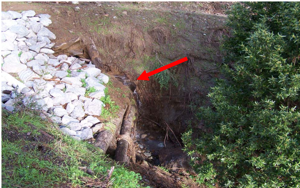
Figure 97: Sunset Trail crossing of small ephemeral creek below Castle Drive erosion site in 2006. Logs indicate this is an historic Humboldt crossing from logging days. Despite rock and plastic pipe, water is flowing along right side of crossing and eroding slope. Humboldt crossing is failing and not able to support rock dumped on it as part of ineffective repair.
