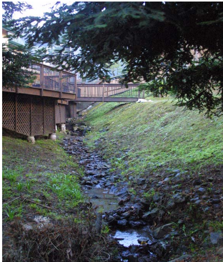
Figure 89: Lining creeks with cement or rock riprap to reduce erosion can result in storm flows undercutting or going around the improvement.
