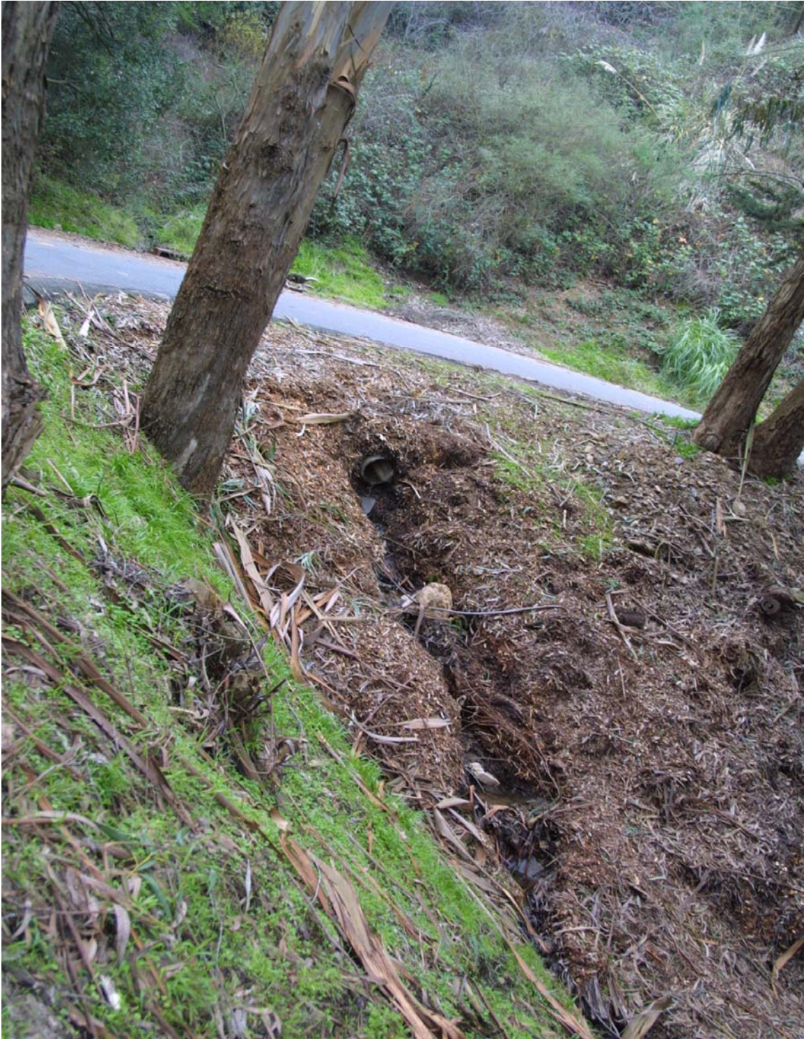
Figure 85: Erosion at storm drain outlet where concentrated flow is released onto the slope without a rock energy dissipater.
