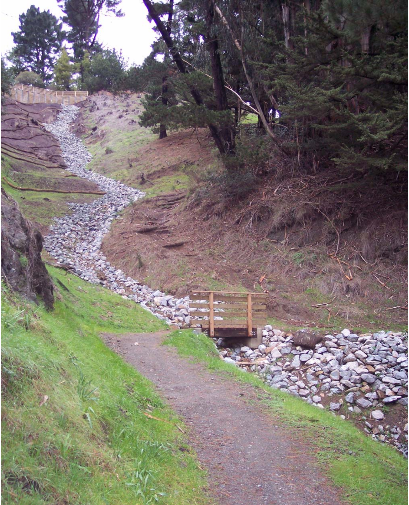
Figure 98: After over 10 years of erosion and several ineffective repairs, an engineered repair was implemented in 2008. Flow was placed in a pipe and buried in rock which fills the gully.
