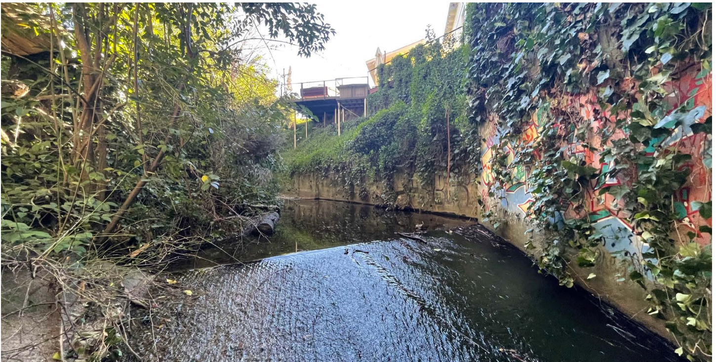
Figure 3: Open section of creek at upstream end of park, facing upstream
