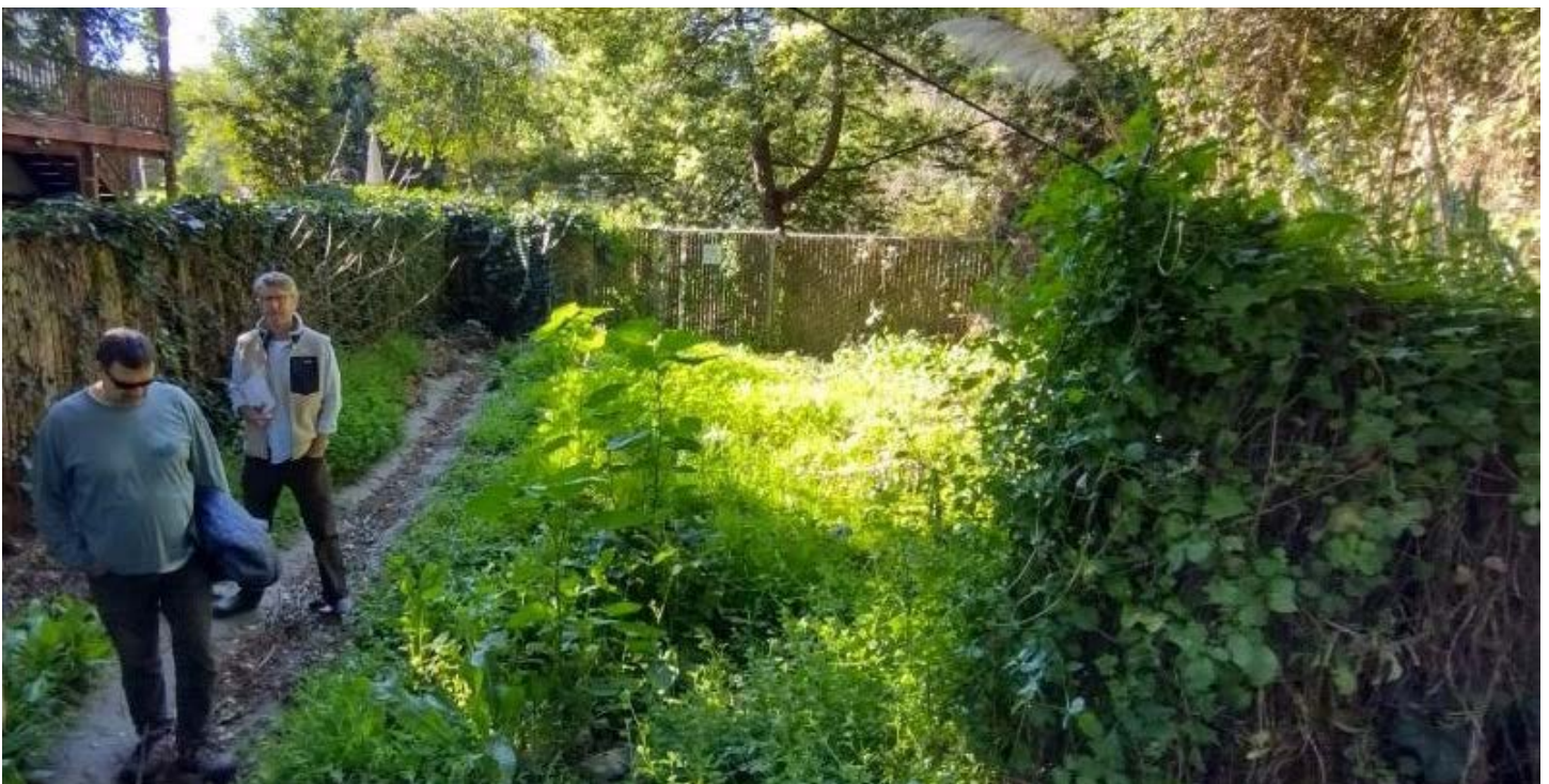
Figure 10: Proposed location for overlook, at downstream end of culvert/swale (creek daylights just past fence in center of photo)
