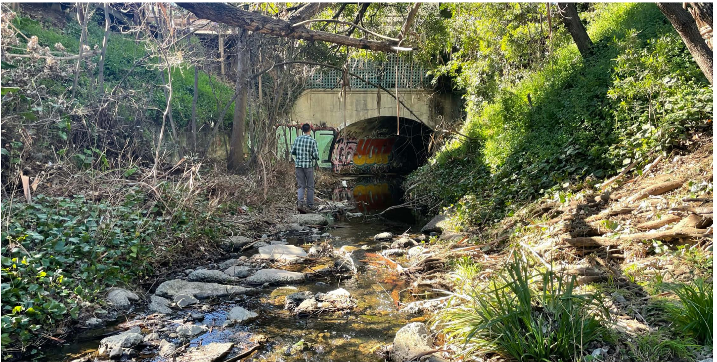
Figure 13: View looking downstream in Sausal Creek to 27th Street culvert
